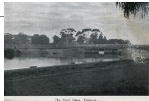
First flood gates at Sawtells Inlet
