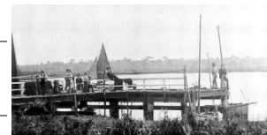
Jetty at Sawtells Inlet
